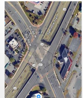
US 29/Rio Overpass
